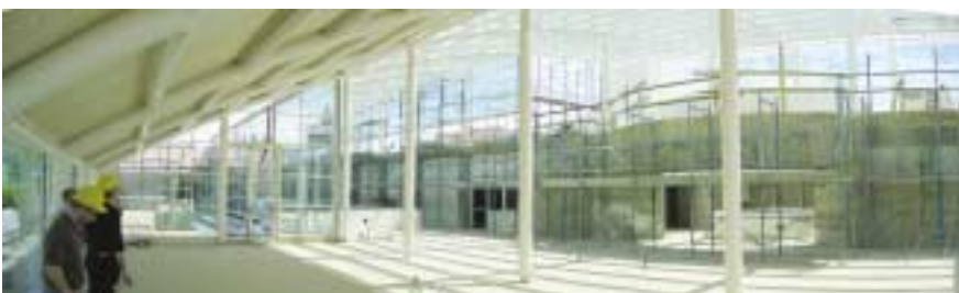
View of the buffer space
