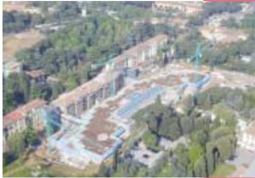
View of the building site
