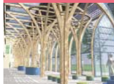
Meyer Children's Hospital, Italy
