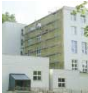
Main building is renovated
