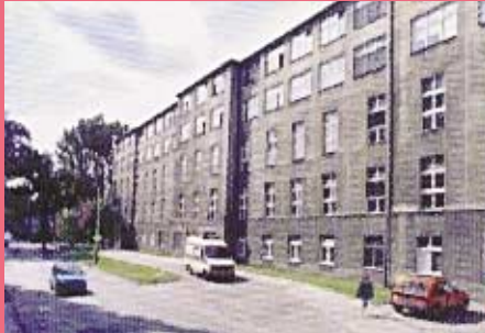
Before renovation from the street
