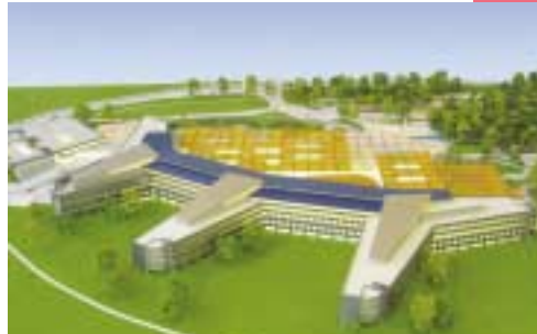
Deventer Hospital seen from the north
