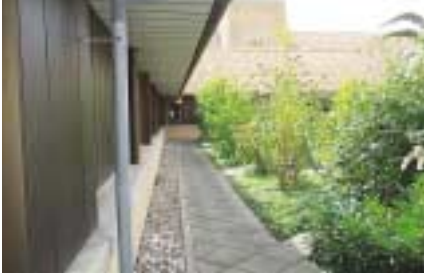
Courtyard before renovation
