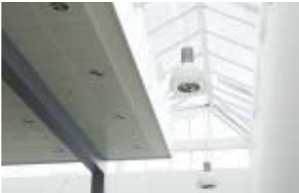
Roof lights for courtyard
