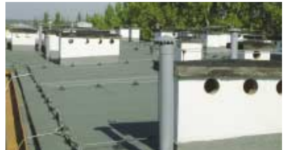
Roof of the main building with the natural ventilation ducts
