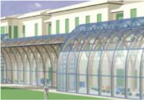
External view of the greenhouse
